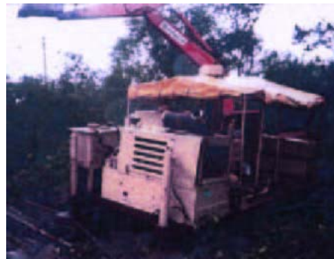
20T Hitachi Tracked CPT Rig on soft ground conditions
